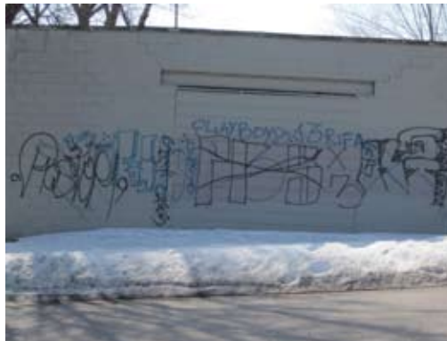
Graffiti is the most visible evidence of gang activity and vandalism.
