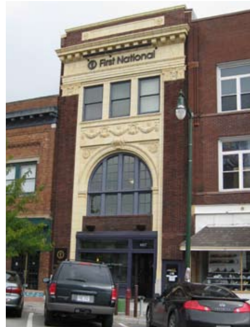
First National Bank restored an 1890s bank building for El Centro Latino de Educación Financiera.
