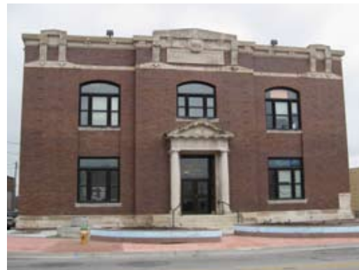
South Omaha City Hall has been restored for office and community uses.
