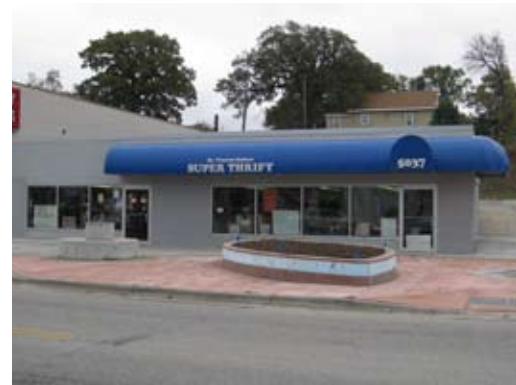
The southern end of the South 24th Street Business District has fewer historic retail buildings.
