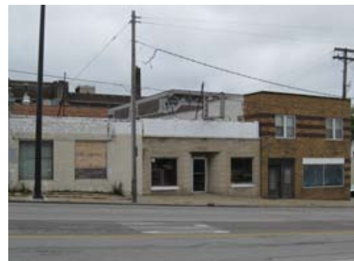
L Street retail renovation opportunity.
